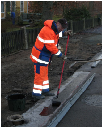
Applying Scan Coat
