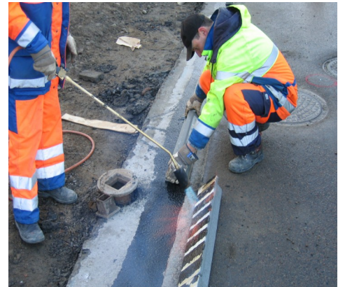
Positioning Scan Kerb
