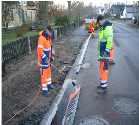
Heating the kerb base
