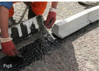
**Scan Kerb alignment**—The kerbs should be aligned using a long wooden handled tool or rubber maul to prevent damage to the kerb face, in hot weather this should be done straight after placement cooler temperatures will slow the process (Fig7).
