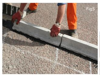
**Scan Kerb base adjustment**—In areas where the highway surface is uneven additional sections of Scan Strip can be used to ensure optimum adhesion, these should be heated prior to kerb placement (Fig6).
