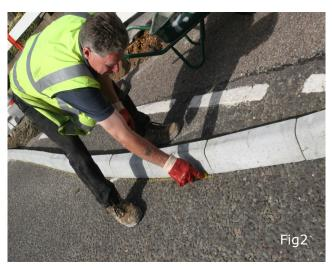
Scan Coat preparation—tip the Scan Kerb forward to reveal the asphalt adhesive coated kerb base. A final sweep of the highway surface to remove any additional dust would be beneficial (Fig3)
